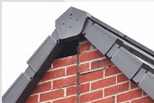
▲ Wall tie failure at gables
