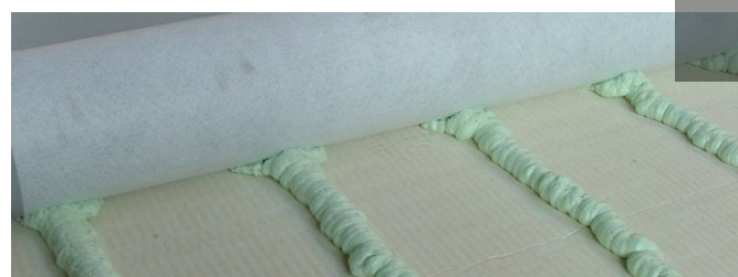
A bonded membrane incorporating HARDROCK® Multi-Fix (DD)
