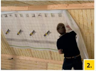
1. Stick Vario XtraFix on a firm surface i.e. Timber Rafters. If necessary, affix additionally at 20 cm gaps 2. Affix the Vario XtraSafe Intelligent membrane against the Vario XtraFix. Lay subsequent strips with a 10 cm overlap.
