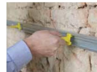
3. Fix plastic clip on horizontal C-channel
